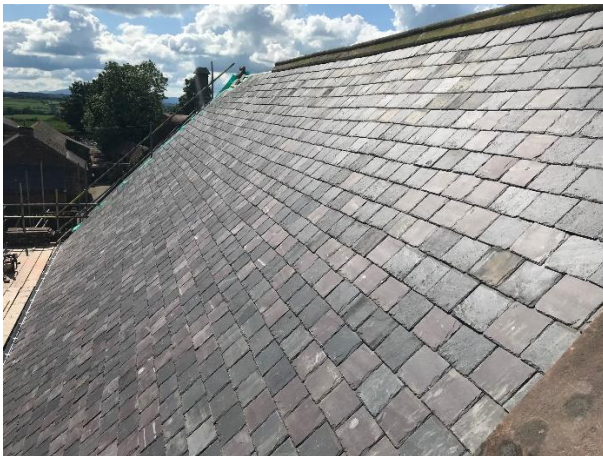
A superb new roof
