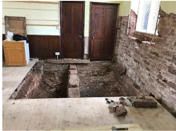
Rotten floor replacement
